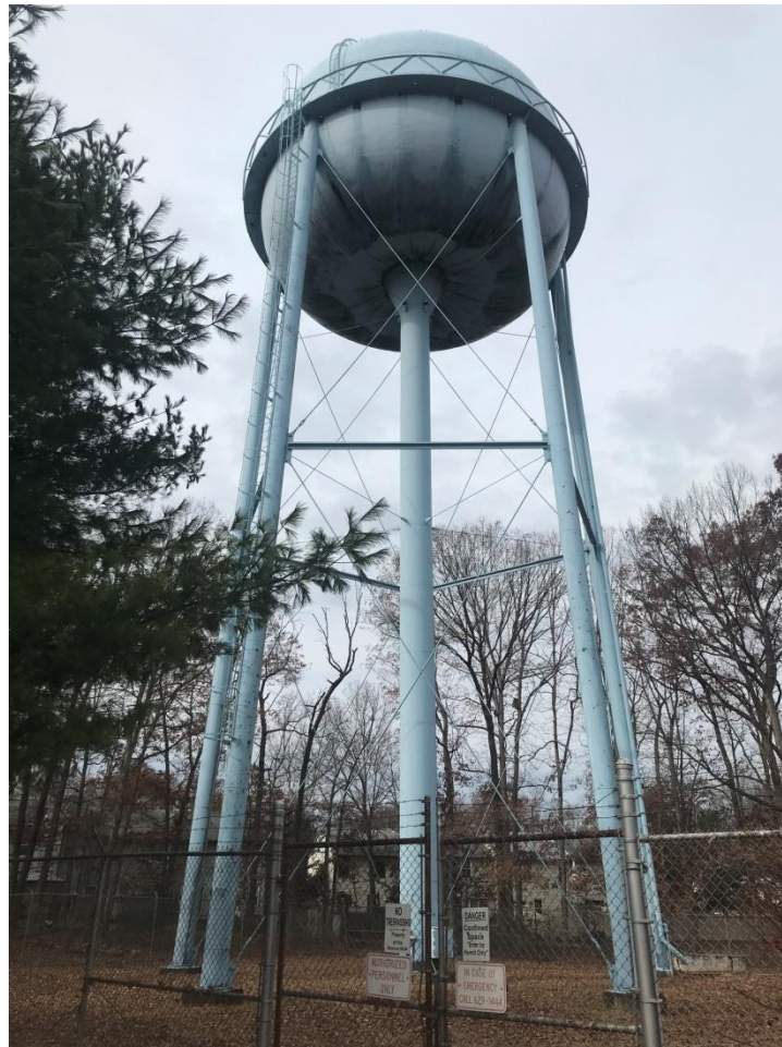
Figure 4: View looking in a northwesterly direction toward the water storage tank located along Herbert Boulevard.
